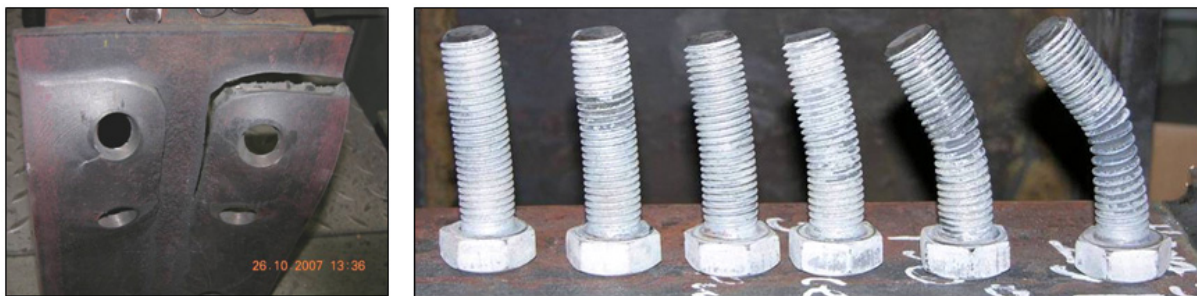
Figure 6: Failure of end-plate connection at 450°C
