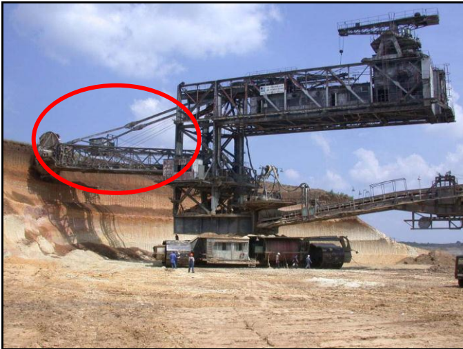
Figure 1 Bucket wheel Excavator SRs 1200
