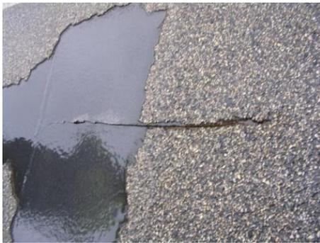
Fig. 5: Longitudinal crack through the deck plate at a stiffener-to-deck plate connection
