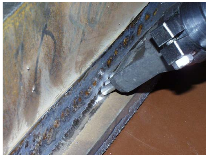
FIGURE 2. The performance of ultrasonic impact treatment.
