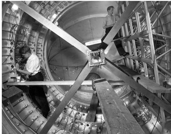
Figure 1. Section of fuselage, 3 m long, being prepared for fatigue testing.
