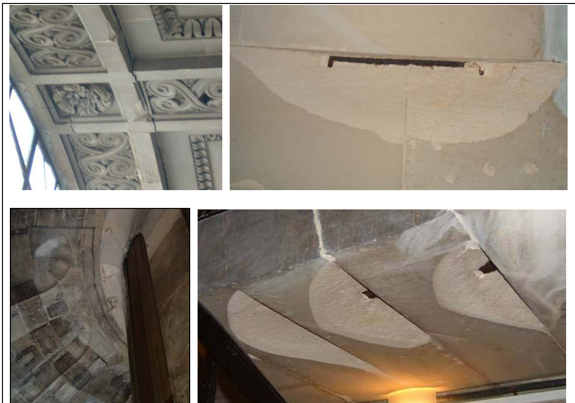
Figure 5: The types of fractures in the stones are very interesting: some are caused by structural disorders, some by the presence of traction in the iron clamps, some by the different thermic behaviour of different parts of the structure.
