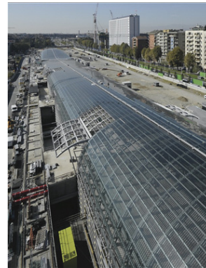
Figure 3: Semi-transparent PV modules used in the shell cover of Porta Susa railway station, Turin, Italy.
