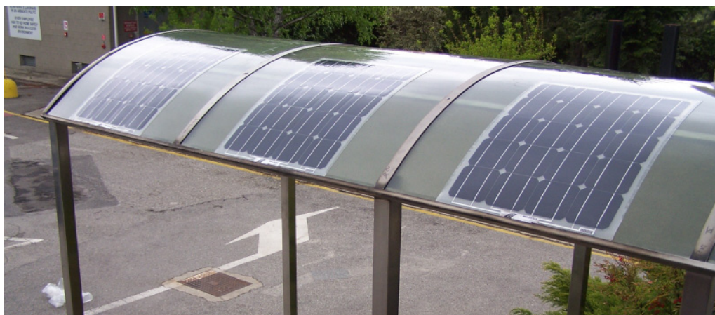
Figure 5: an example of flexible PV modules glued on a curved substrate.
