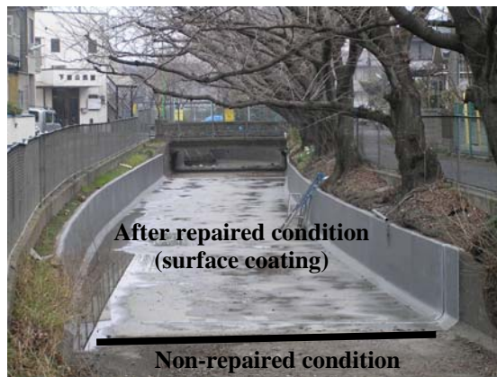
Photo 3 Comparison between surface coating and non-repaired conditions in monitoring water channel.
