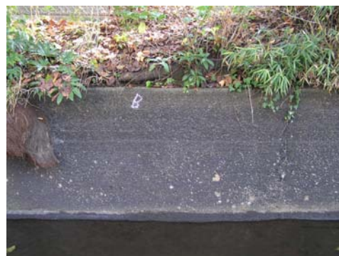
Photo 2 Overview of non-damaged concrete water channel wall in normal section.
