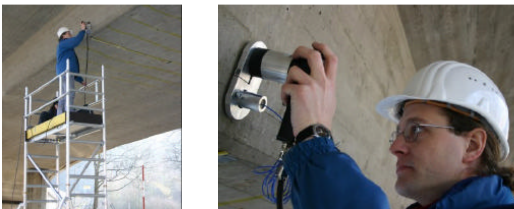
Fig. 3: Void detection using the DAI-1 impact-echo system at a concrete bridge.
