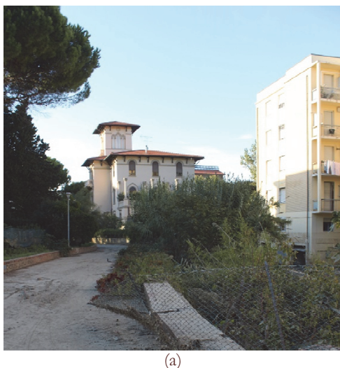
Figure 7: Buildings damaged by the flood, photo taken from an inner street near via Nazario Sauro. Building where the tragedy occurred, on the foreground a small wall overturned by the load of the flow; (a); other blocks of flats, the basement was totally flooded, the overflow reached the windows on the first ground (b).
