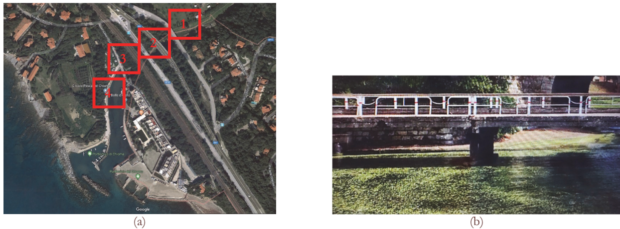
Figure 14: Top view of the Chioma small harbour (a) View of the small bridge with the intermediate pier (b).
