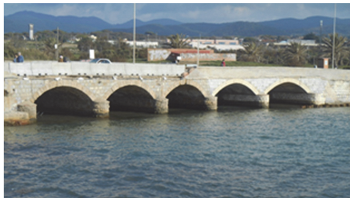
Figure 10: Bridge on the Ardenza river, view from the sea side.
